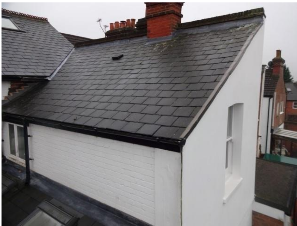
Roof over bathroom bedroom 3
