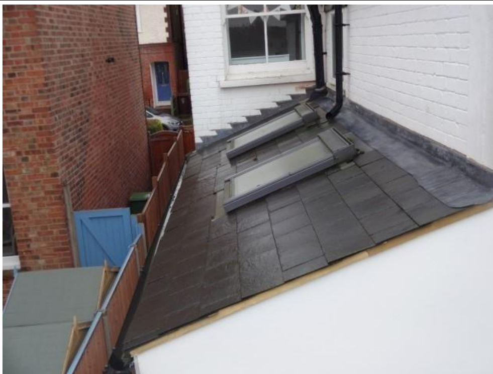
Roof over kitchen
