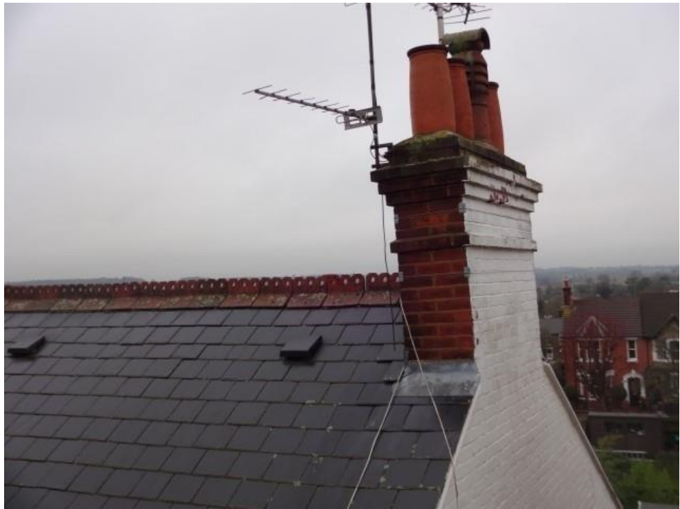
Front chimney stack
