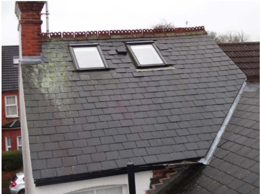
Roof over bedroom 2
