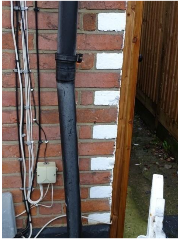
Front gutter down pipe
