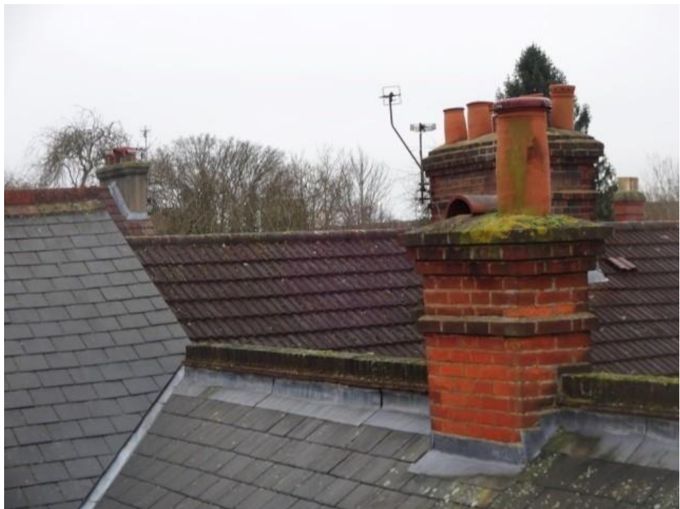
Rear redundant chimney stack
