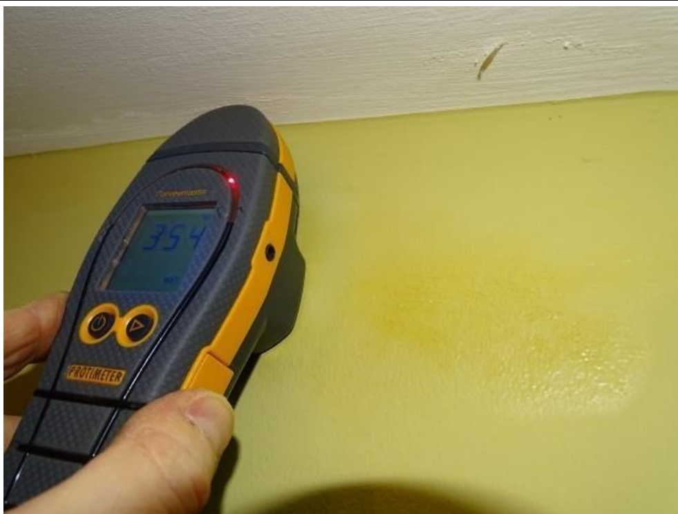
Dining room chimney breast at high level
