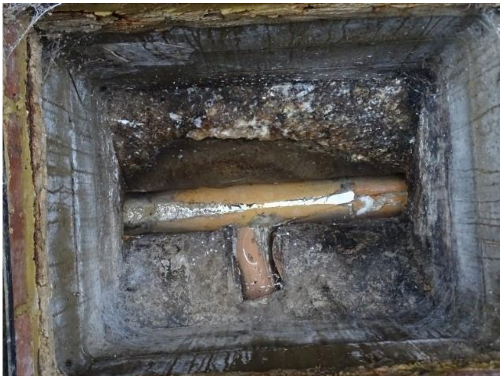
Manhole down alley way
