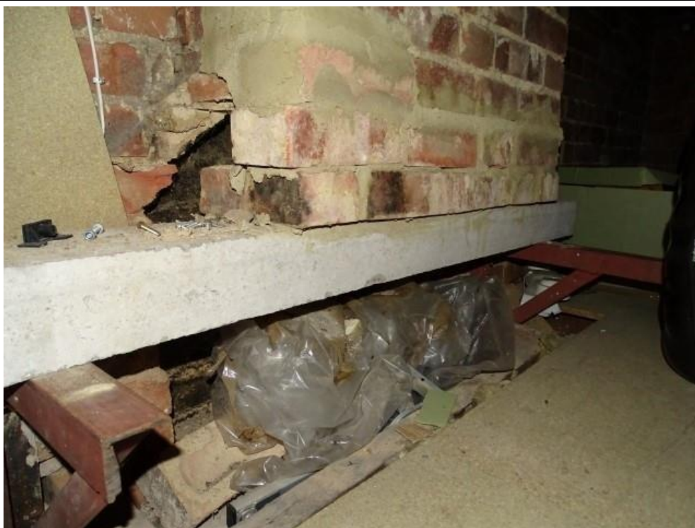
Chimney stack supported in loft
