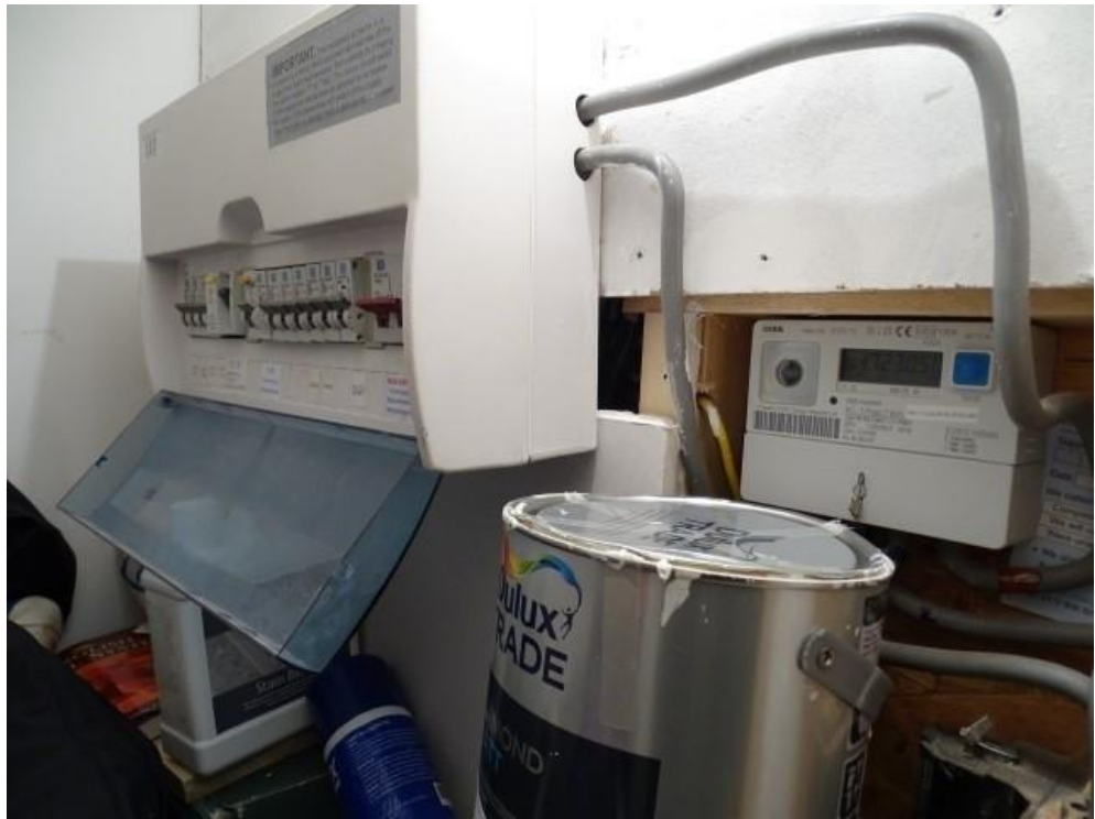
Electric meter and consumer unit
